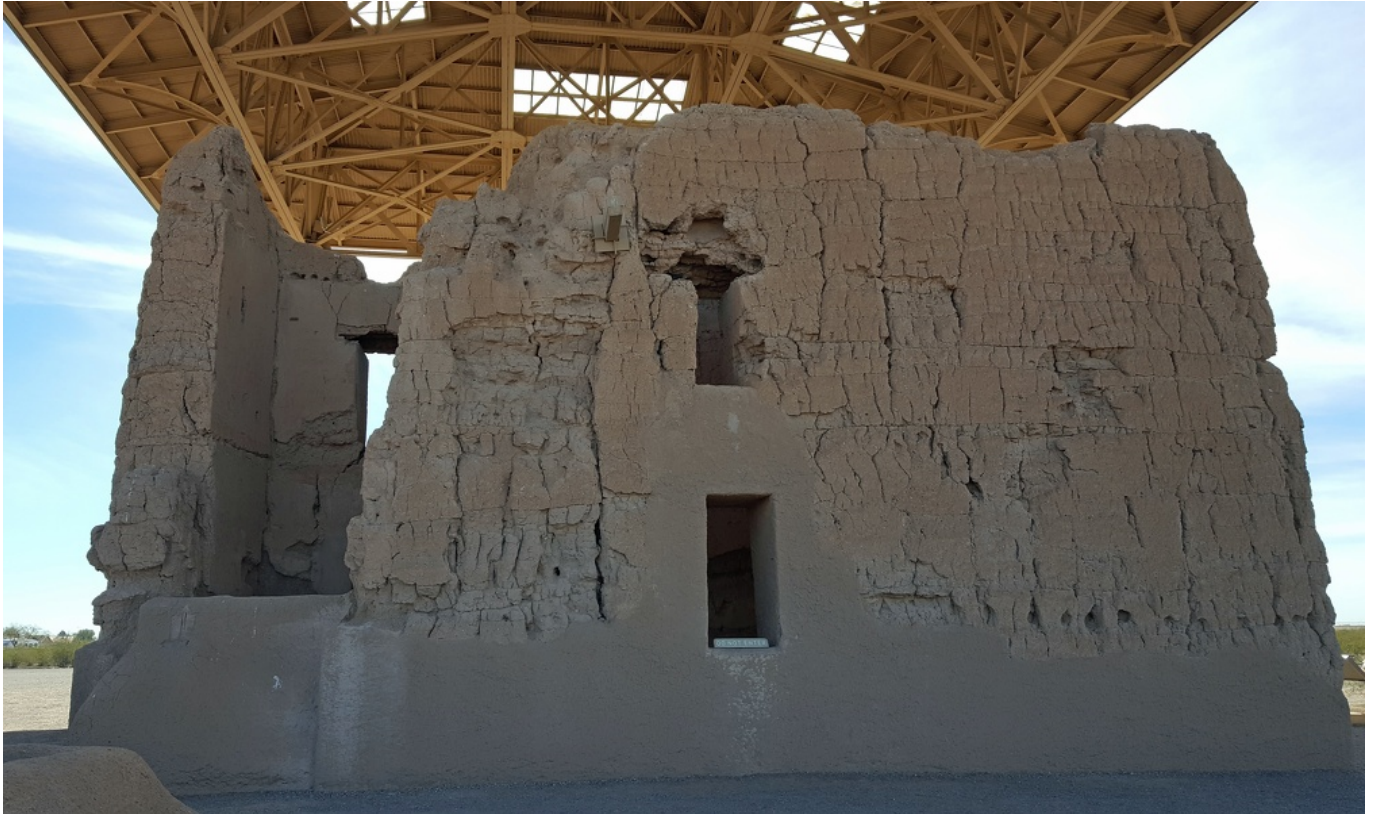
Roof added to help preserve the remaining structure.
